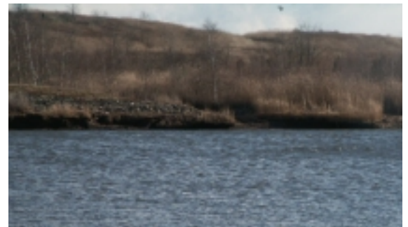
Raritan River lapping the banks of the landfill. The restoration project will stabilize the riverbank, possibly using native vegetation and rip rap.
