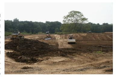
Sadat Associates, Inc. (SAI) was retained by the owner to design a Class III dam to replace the partially constructed dam, to create a pond for fish breeding. The existing earth dam was constructed with residual clayey soils from the underlying shale bedrock formation.
