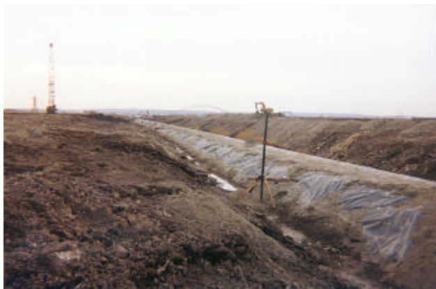
The 5,000-foot culvert was graded to allow tidal flow to enter an upstream tidal pond and also accommodate maximum freshwater inflow.
